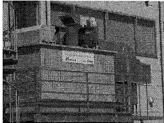
Fig. 6 Appearance photograph of New Desiccant Air-conditioning System
