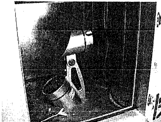
Fig. 9 Photograph of Enumeration of Airborne Microorganisms (Inside of Supply Air Duct)
